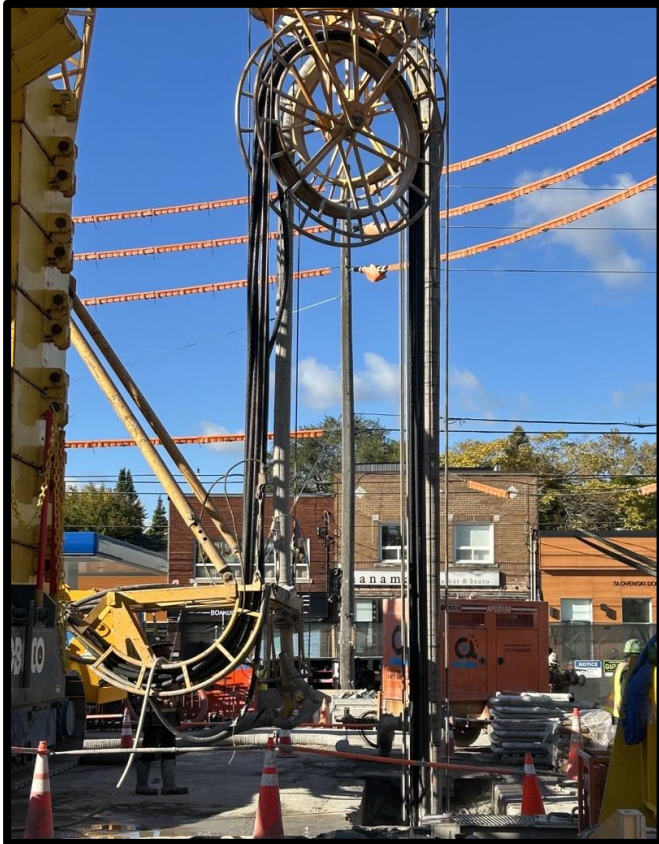
Excavating panel at Sammon
