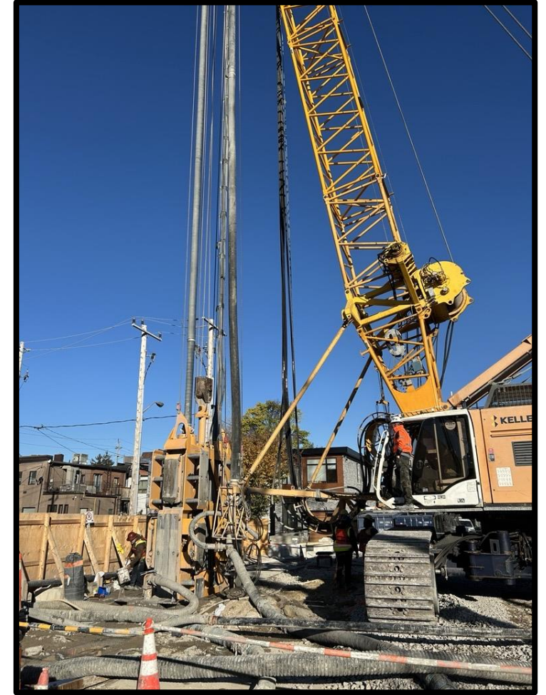
Excavating panel in Pape north shaft
