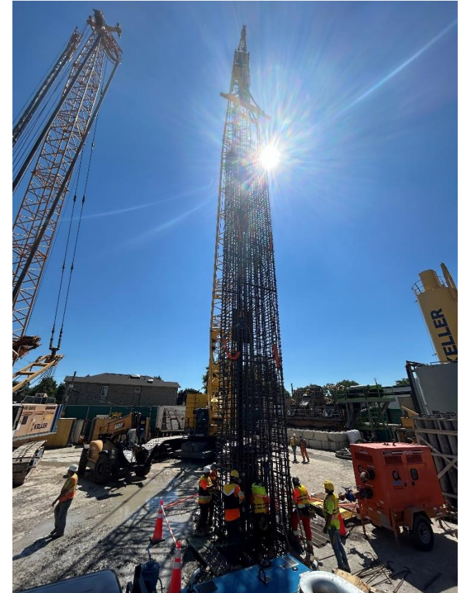
Carefully placing a rebar cage into the excavated panel
