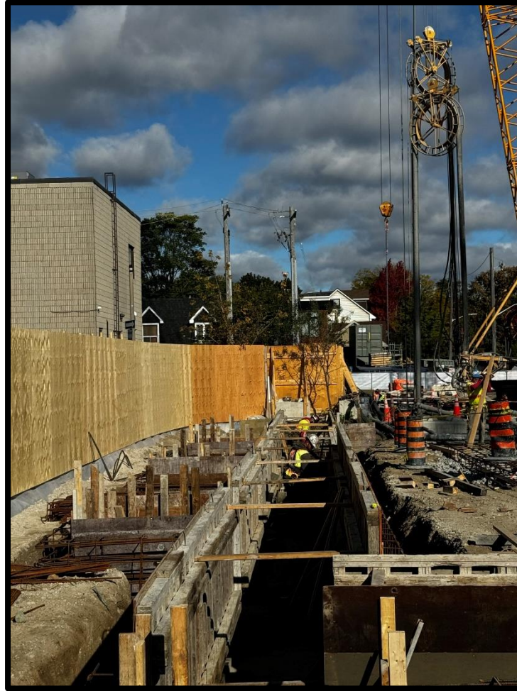
Building Pape north guidewall
