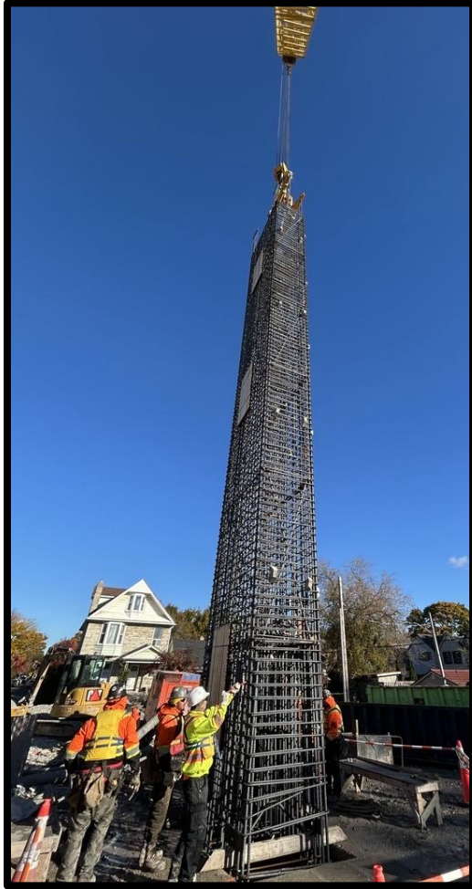
Lifting a rebar cage before inserting into excavated panel
