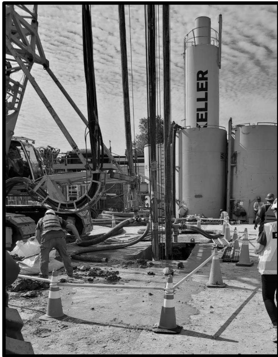
Excavating a panel with the hydromill
