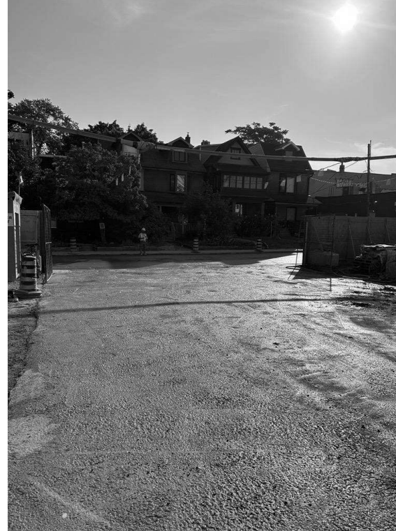
Concrete pad at the Eaton Gate
